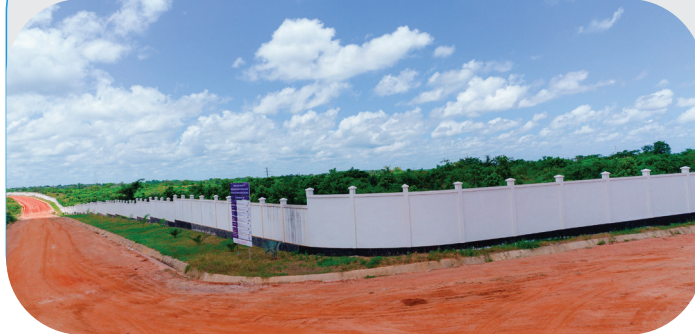
9 km boundary wall completed with 2.5 metres height and 9.1 km road around the wall
